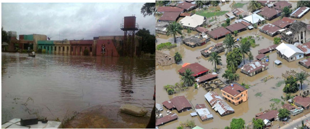
Fig 1. situations during the 2012 flooding in part of the study area
