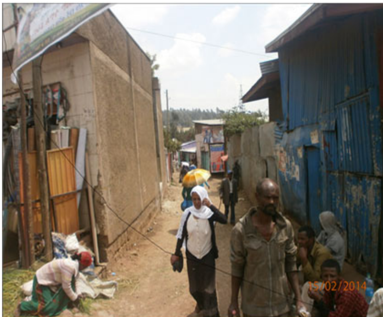
Figure 5.15 Narrow Foot Paths: Too Narrow foot Paths make walking uncomfortable and unsafe. When Two building enclose this narrow space due to absence of side set-backs
