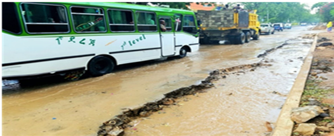
Figure 5: Flooding to both the right and left side of the drainage system
