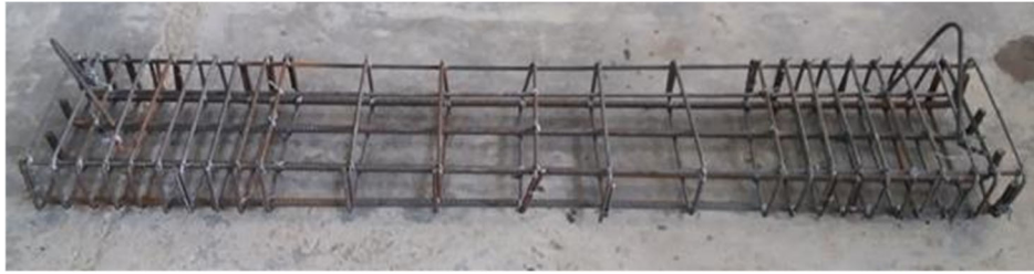
Figure 1. Steel reinforcement cage
