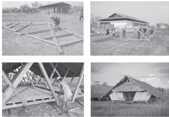
Figure 9. Safe and straightforward temporary housing built with locally available materials by the local workforce, assembly, and maintenance are accessible because users know the building techniques and materials. Source: (Félix et al. , 2013)
