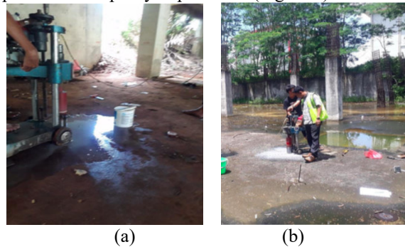
Figure 1. Basement condition: (a) protected, (b) unprotected
