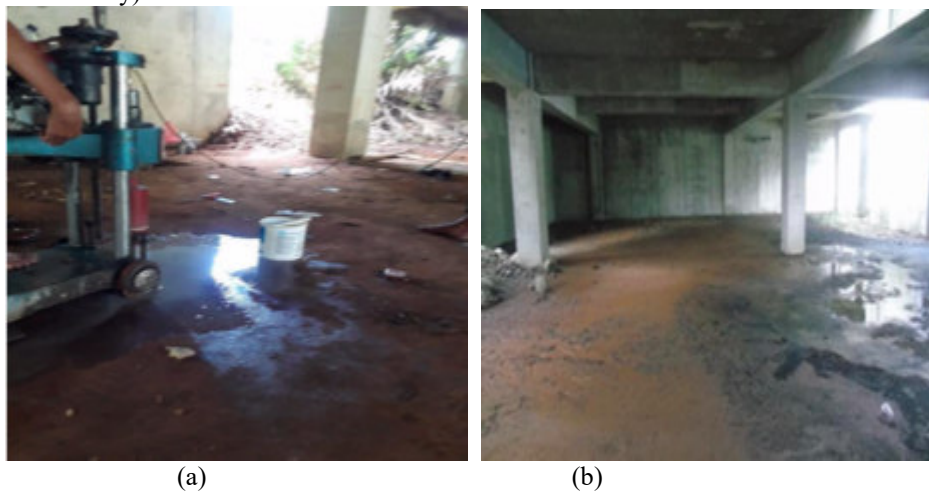
Figure 1. Concrete condition: (a) Protected concrete, (b) Concrete submerged in mud
