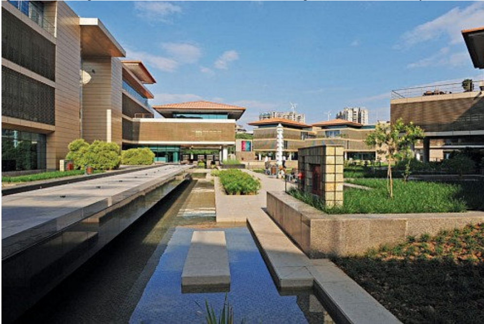
Figure-1 Suzlon One Earth Building, Pune – LEED Platinum and GRIHA Certified 3
