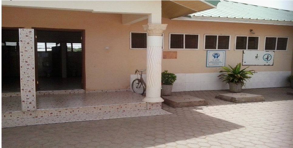
Plate 3.0. Shows the clean entrance of a POMPT (WC toilet) in Kpaguri area. The floor tiles are clean with no flies.
