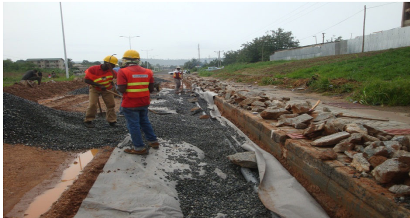
Fig 2: Use of geotextile material at ch 880
