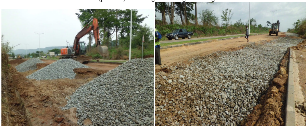
During remedial works (Placement of crush rock base material)
