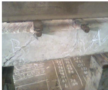
(b) Crack progression
