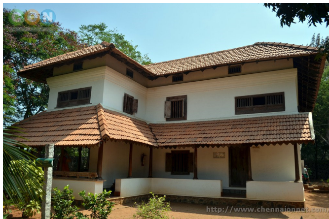
Figure 1. The Recycled House, build 2007 (Chennai.)
