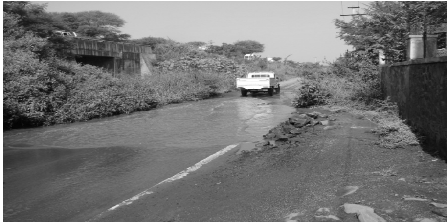
Figure 1: Road under water near Punawale village
