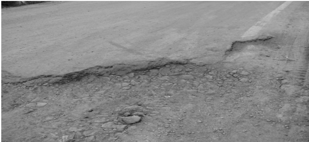
Figure 3: Stripping of bitumen
