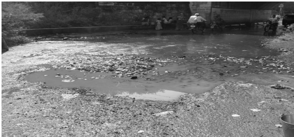
Figure 10: Road affected by flow of water
