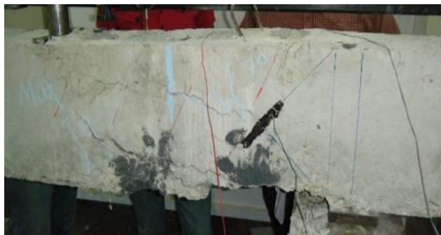
Fig. 9. Crack Patterns of Specimen S-IER
