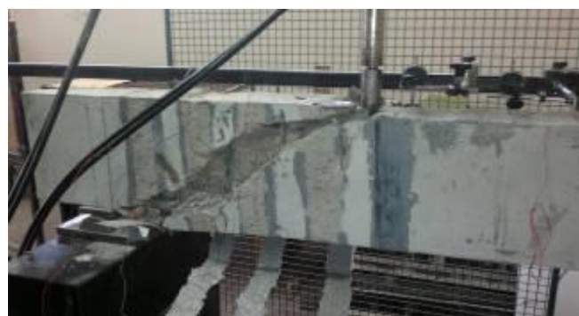
Fig. 8. Crack Patterns of Specimen S-EBR
