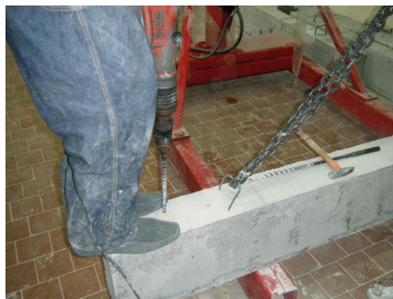
Fig. 2. Drilling of Holes for Specimen IER
