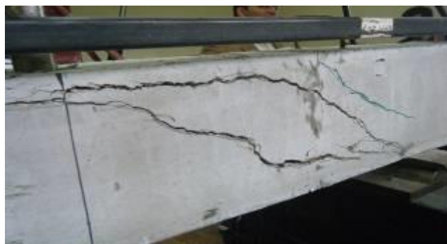
Fig. 7. Crack Patterns of Control Specimen
