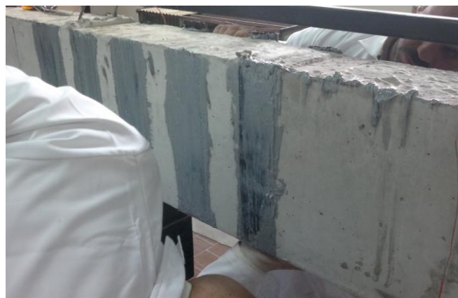
Fig. 4. Strengthening of Specimen EB
