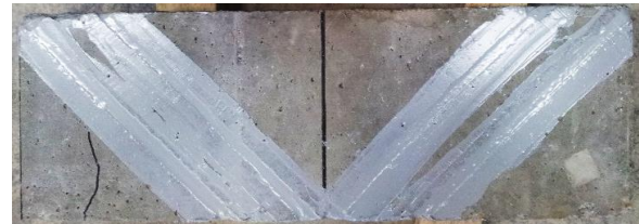
Fig. 6.a A1T-SB after repairing in shear.
