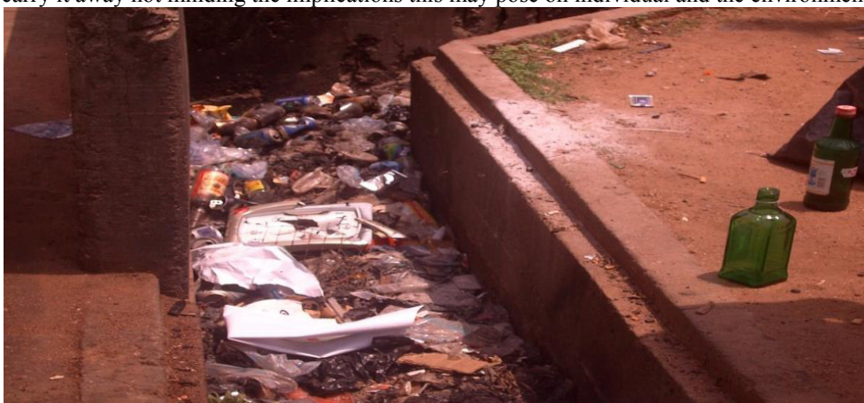
Plates 4a, Dumping of waste inside gutter – an indecent method of disposing waste
