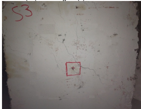
Figure (4) Failure Mode of Panel (S3)
