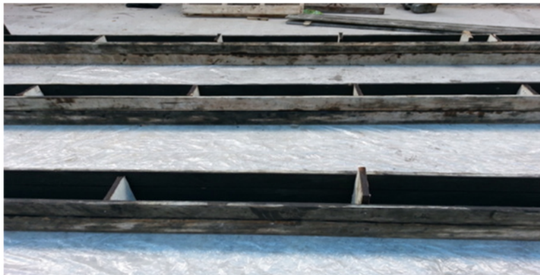
Figure 4. Wooden Formwork of Specimens
