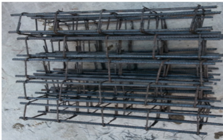
Figure 5. Steel Cage of Specimens
