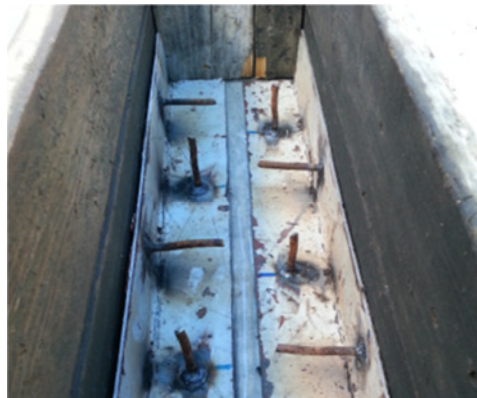
Figure 10. Steel Angles with Connections in Formwork
