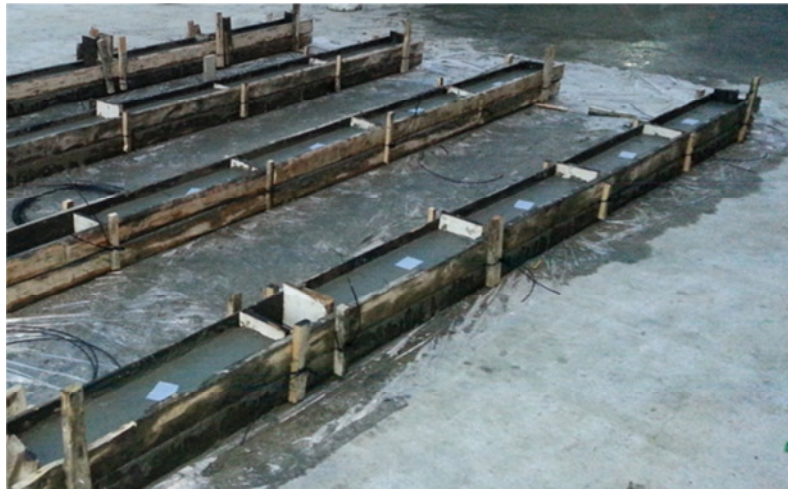
Figure 6. Casted Concrete in the Formworks
