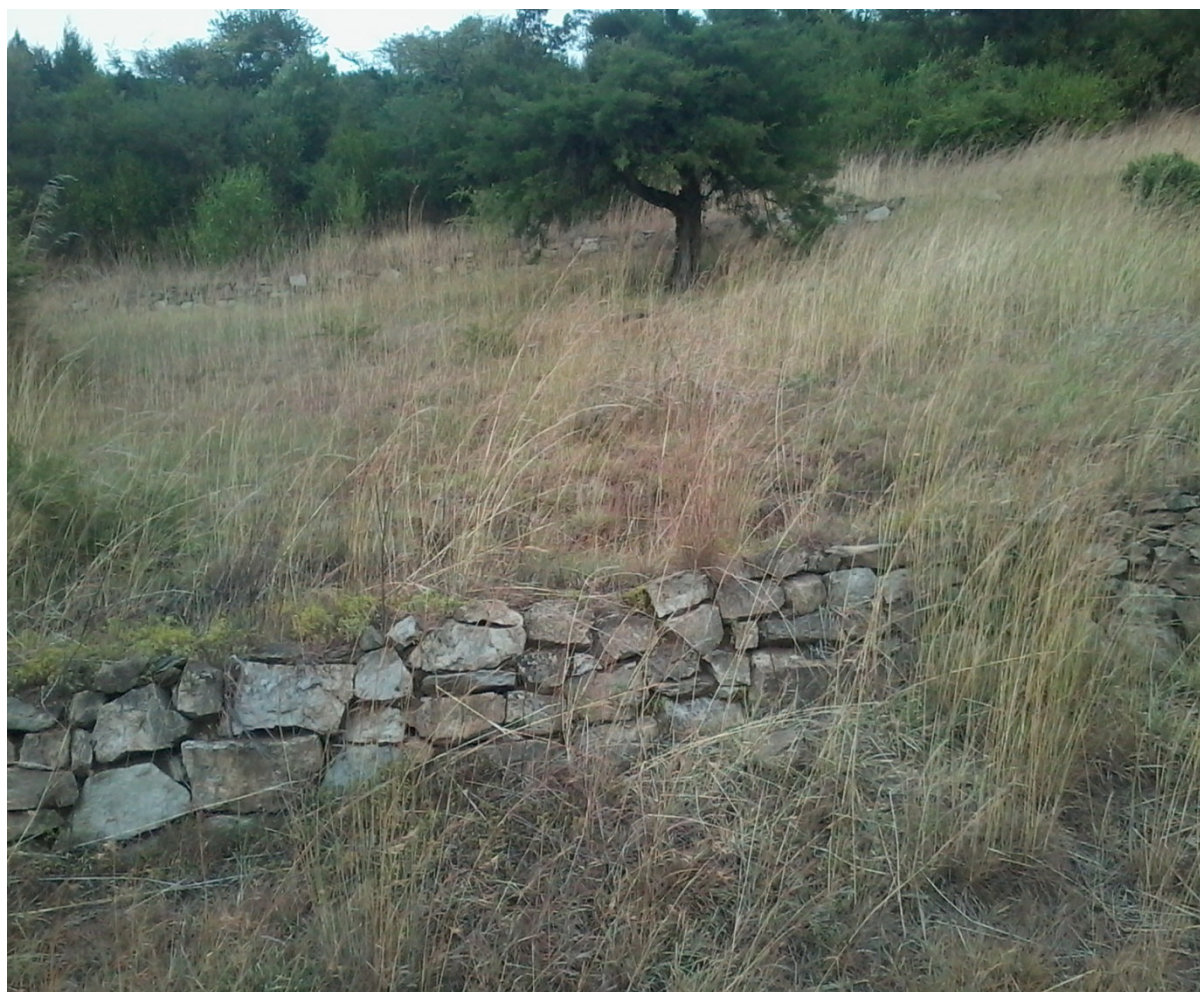
Figure 3. Wadesa (Chiro area) community based watershed developments partially
