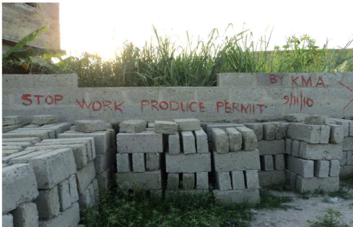
FIG. 4.3 a & b. Warning Inscription, “Stop Work Produce Permit” Or To Be Demolished Due To Flouting Of Building Regulation.
