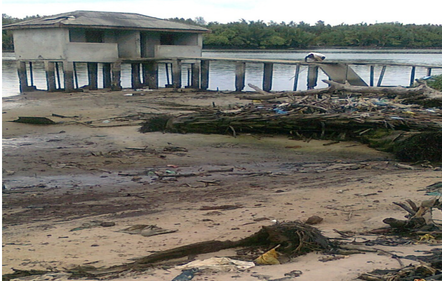
Figure 4 The traditional “Pier Toilet” common in Waterside settlements in the city
