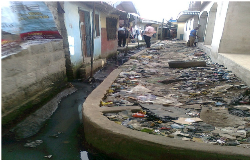
Figure 6: Water is always stagnant in the few available drains in waterside settlements with sickening sight and offensive odour. The use of domestic waste for land filling is a common tradition in waterside settlements.
