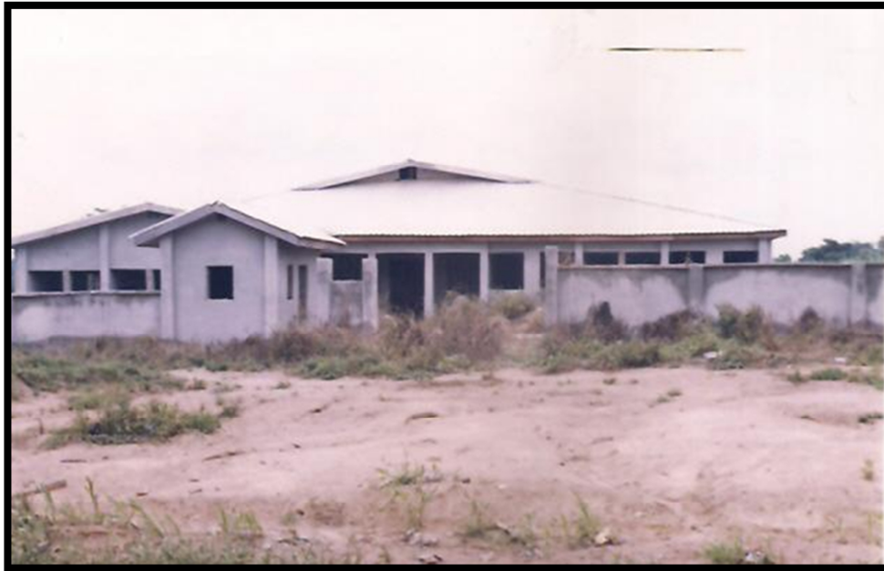
Plate 3: On-going Hospital by Government
