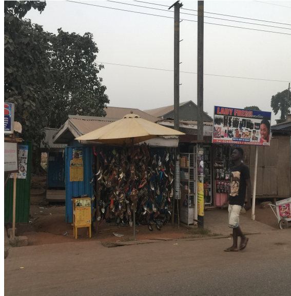
Figure 4: A Container structure as footwear shop at Abuakwa-Kumasi along the Kumasi-Sunyani main arterial road (Source: Authors', 2015).
