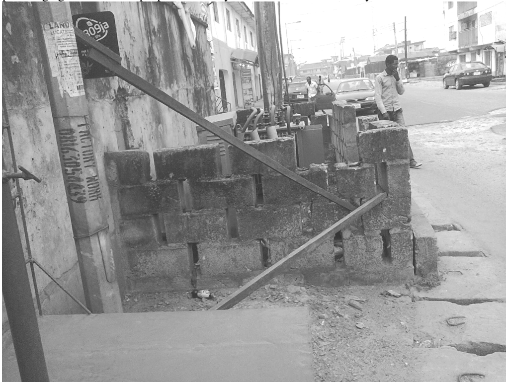
Figure.5 Electricity transformers are located indiscriminately by the Power Distribution Companies in the cities without any regard for environmental safety and planning standards
