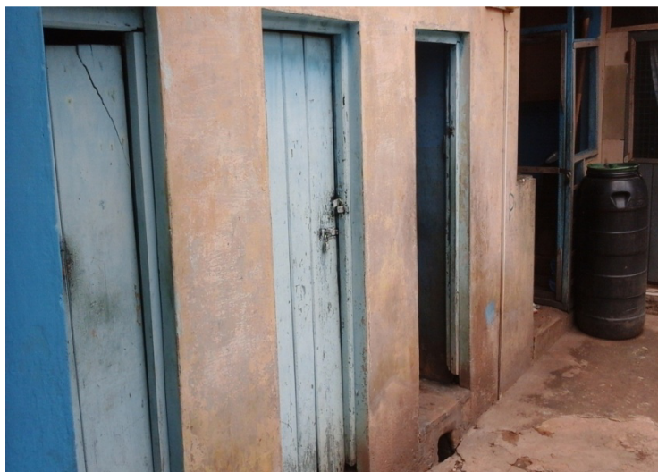
Figure 5: Bathroom in one of the compound houses in the selected neighbourhoods Source: Field Survey (2015)
