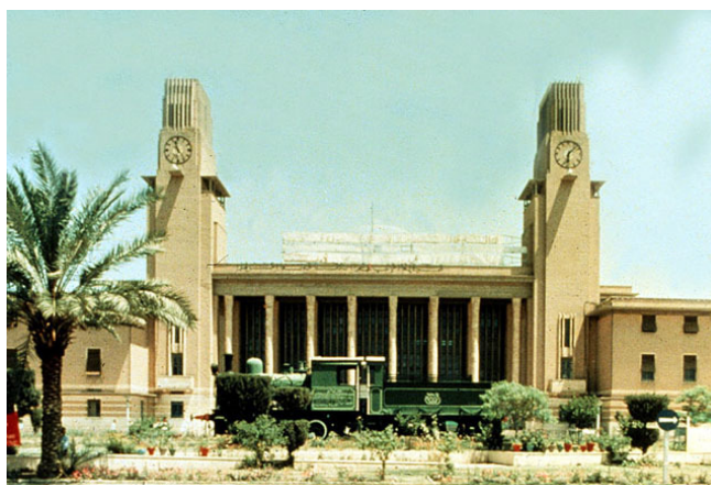
Figure 7: Baghdad's Rail Station
