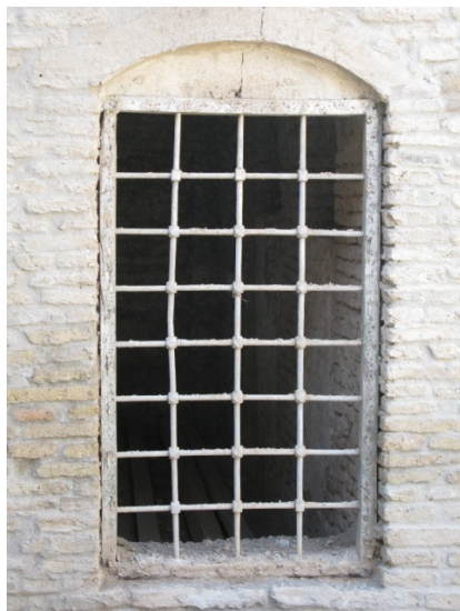
Figure 17: A Typical window
