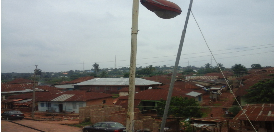
Plate 1: showing unorganized buildings without access due to lack of approved layouts in Ifon.
