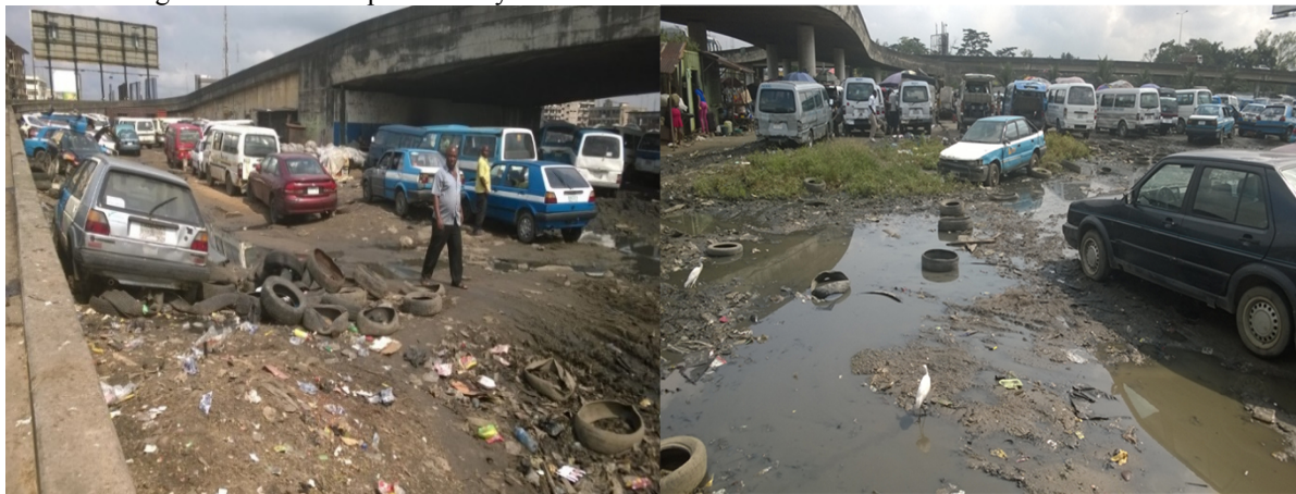
Picture 1: Abuse of Road Infrastructure
