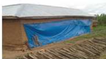
Plate V: Dry flood proofing with waterproof sheet Source: Authors' Field Work 2013
