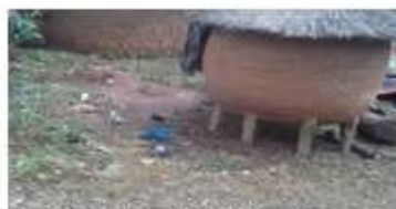
Plate II: Raising the building above flood level with short mud piles Source: Authors' Field Work 2013
