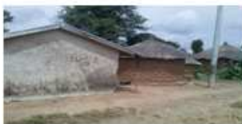
Plate IV: Plastering mud wall with sandcrete mortar Source: Authors' Field Work 2013
