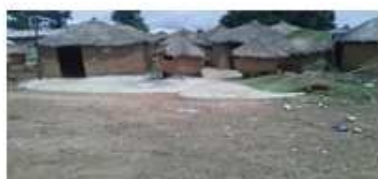
Plate VI: Concrete Apron around mud wall bases Source: Authors' Field Work 2013
