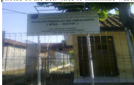
Figure 1. Installing a Wastewater Treatment Plant (WWTP) in the Kauman Village
