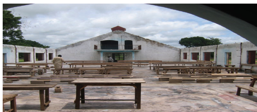
Plate 7: A Big Church Burnt in Jos North, (Field Survey, 2011)
