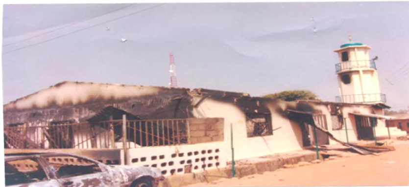
Plate 2: A Mosque Burnt in Jos South, (Field Survey, 2011)
