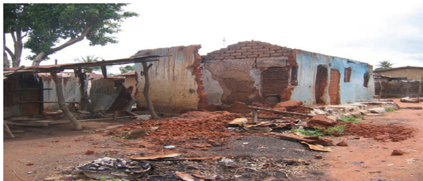
Plate 11: A House Devastated and Destroyed in Jos North, (Field Survey, 2011)
