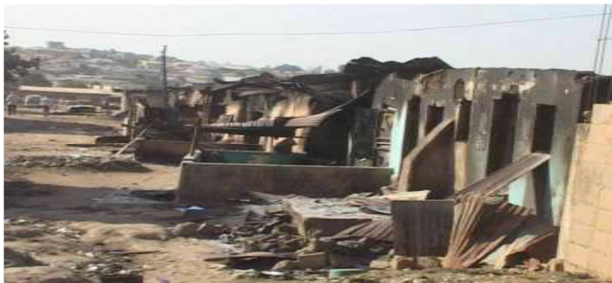
Plate 5: A Neighbourhood Burnt in Jos South, (Field Survey, 2011)
