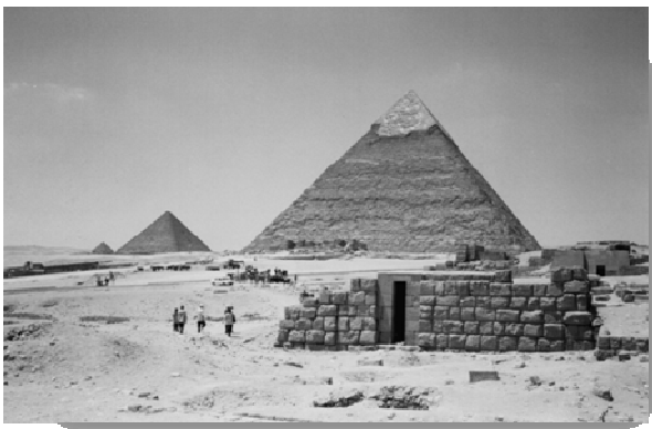
Figure (2) The remains of the limestone coatings of the Pyramid of Khafre .
