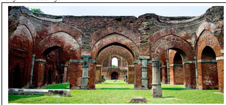
Darasbari Mosque (before reconstruction): Chapai Nawabgang
