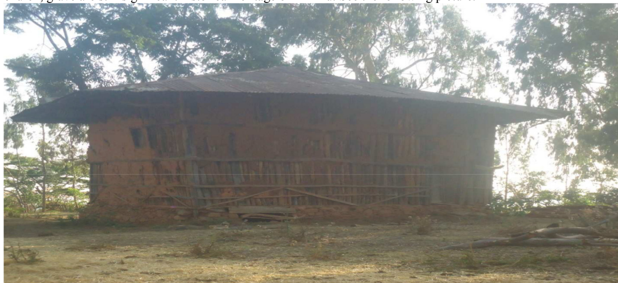
Figure 1. Fitawräri Duguma Jaldeso's Palace, constructed in 1930 E.C/1938. Photo taken by the author, February, 9, 2013.
