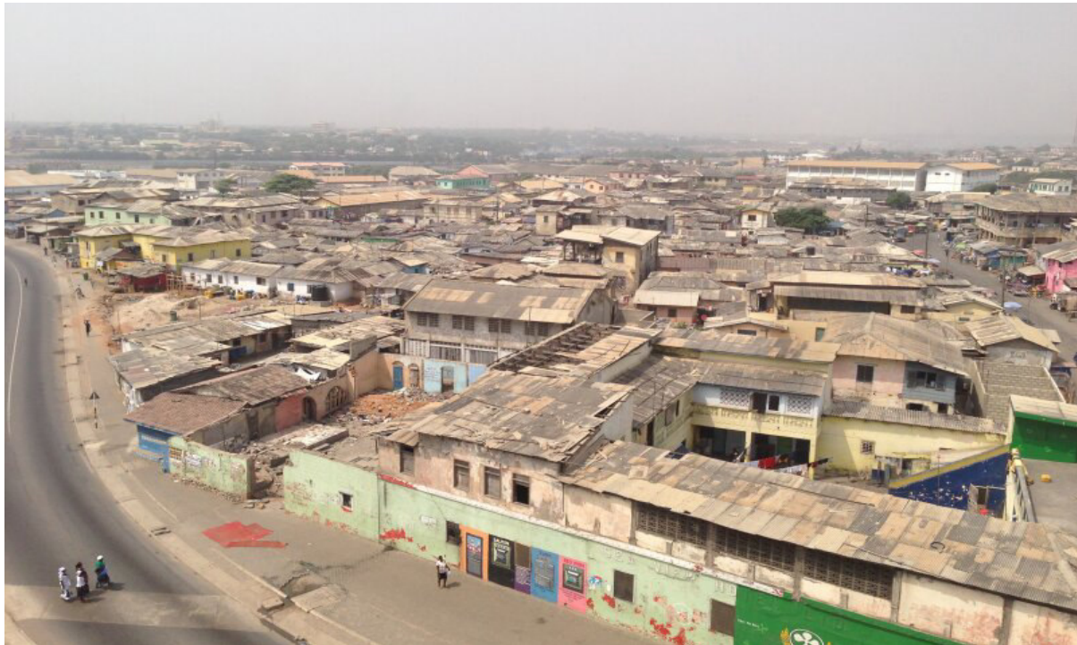
Figure 2. Aerial view of part of Ga Mashie/Old Accra, showing the common two-storey properties and generally worn-out and blighted properties, with highly rusted roofscales. Source: Google maps.com, 2021
