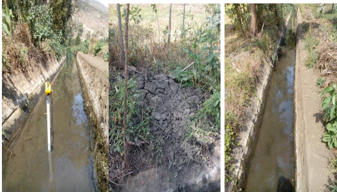
Figure 7. Measuring depth of sediment deposited in canal
