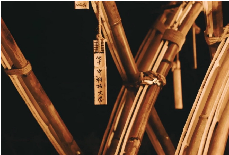
Figure 14. Close-up showing the interconnection between arches, illuminated artificially at night. Photograph: Tan Gangyi
