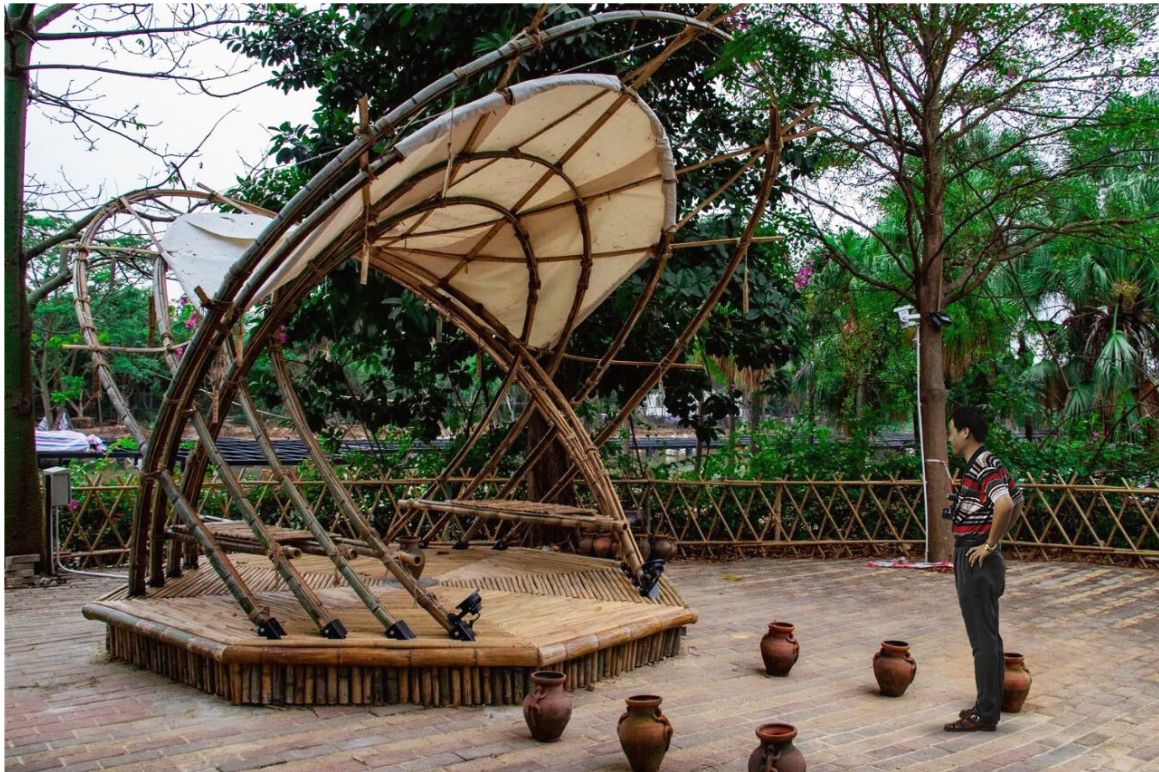
Figure 4. Built prototype of the Wing pavilion during the presentation day. Photograph: Tan Gangyi.
