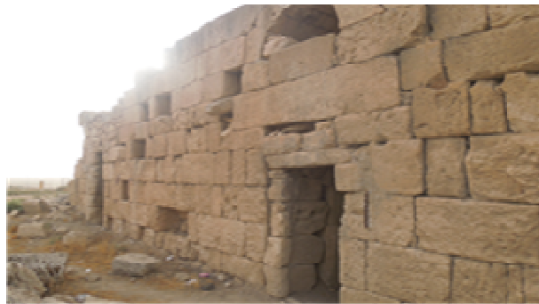
Figure 5. An inner load-bearing wall showing the stone blocks and mortar joints
