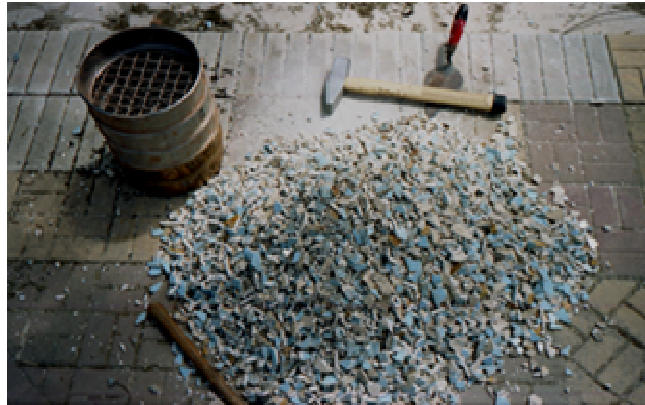
Figure 4. Crushing the broken bathroom tiles to proper sizes.
