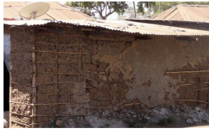
Plate 1: Bamboo Reinforced Mud-wall Source: Anon, 2012.
