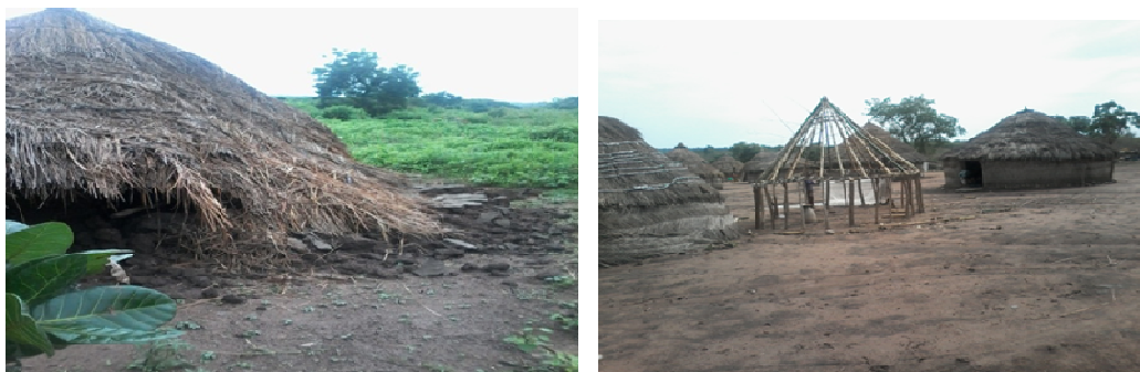
Plate 3: Collapsed Structure During Heavy Rainfall and Typical Structure Under Construction at Gaa Bororo, Ogbomoso North Local Government Area, Ogbomoso. Source: Author's Fieldwork, 2015
