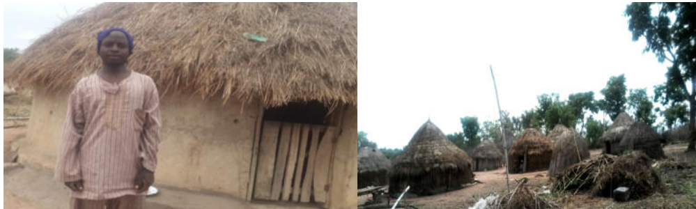
Plate 1: Indigenous Fulani Housing Type at Gaa Oguro-ologurun, Ogooluwa Local Government Area, Ogbomoso.
