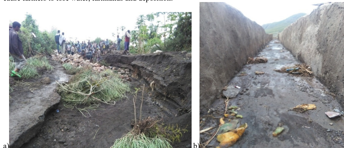
Figure 4. Earthen (a) and cemented canals (b) at Weynalem scheme Source: Photo February 20, 2018.
