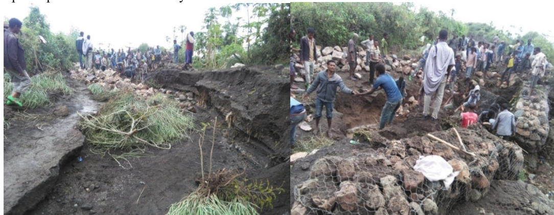
Figure. 2. Operation and maintenance work in diversion Beles at weynalem scheme
