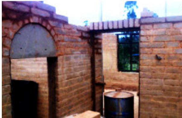
Plate 11: Compressed earth blocks for wall made from the mixture of cement and laterite. Source: Opaluwa et al., 2012.
