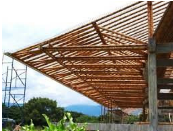
Plate 8: Bamboo as roof structural members
