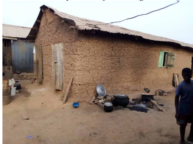
Plate 1: Reddish brown surface of a wall constructed with laterite: Authors Field work, 2019
