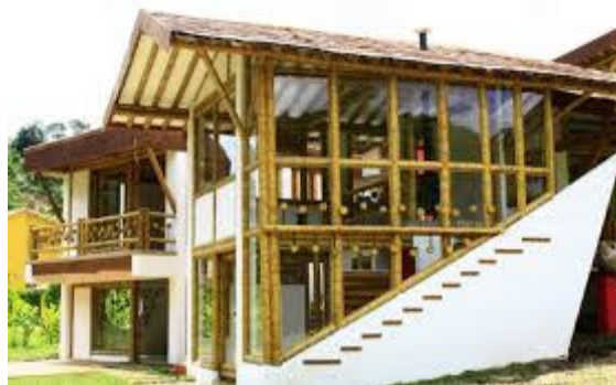
Plate 7: Bamboo as fabric and structural support for building. Source: MT Bamboo Plywood, 2020
