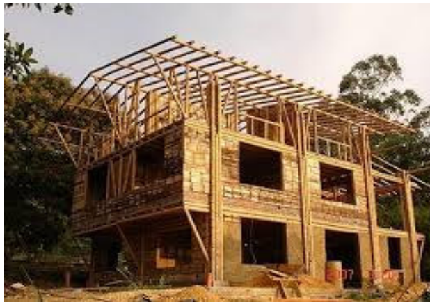
Plate 9: Bamboo as roof structural members and column supports
