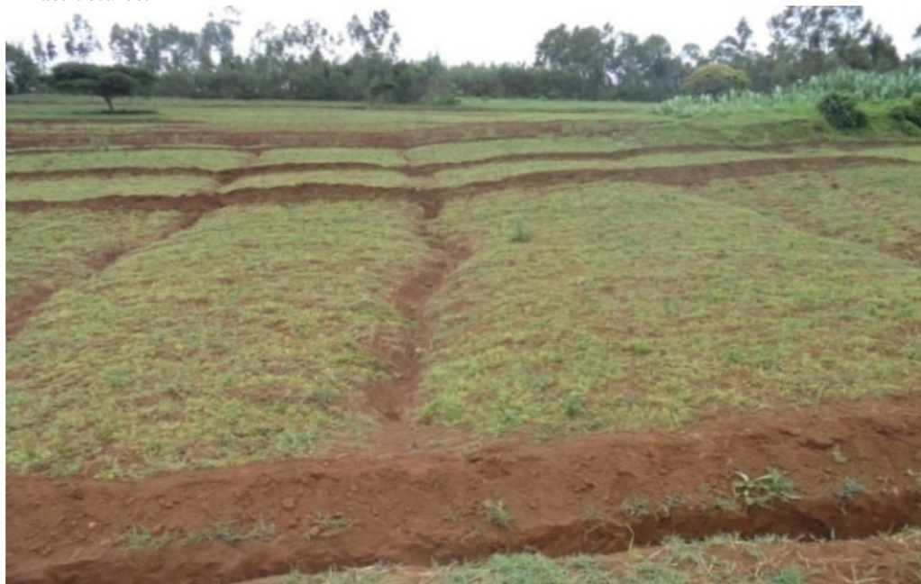
Figure 17: Broken SWC structures that exacerbating soil loss in the Upper part of the study area (Photo by Abebayehu in July, 2013).
