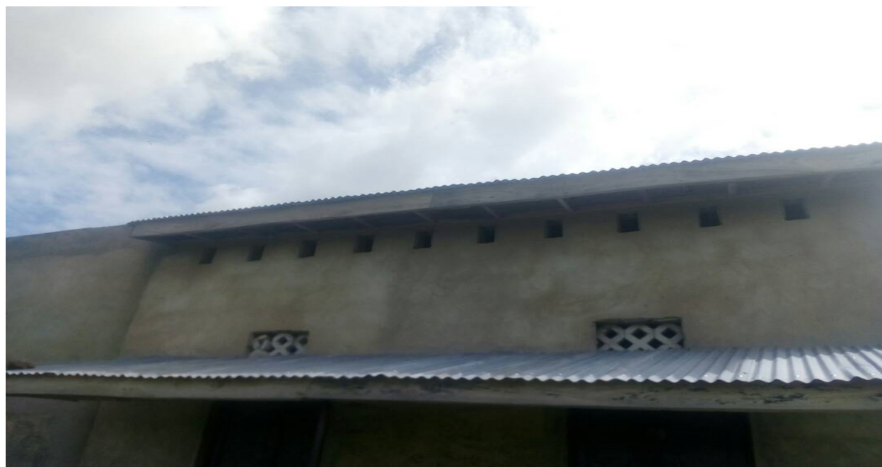
Plate 3: Onion Storage at the Top of the roofing
