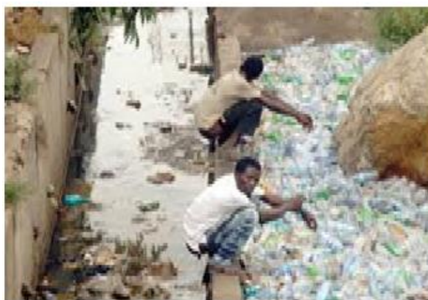
Figure 1: People practicing open defecation and polluting underground waters
