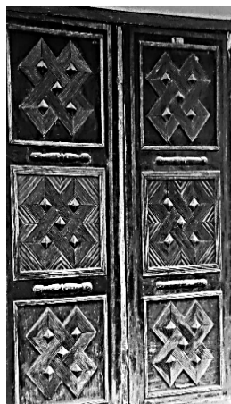
Figure 17: Door adorned with tar-rod forming a guilloche design (Photo: Abejide, 2019).
