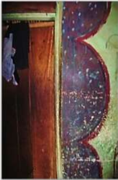
Figure 3: Inner portal of No. 21 Aládiye Street, Òsogbo decorated in synthetic paint (Photographed by F. M. Abéjidé, 2018).
