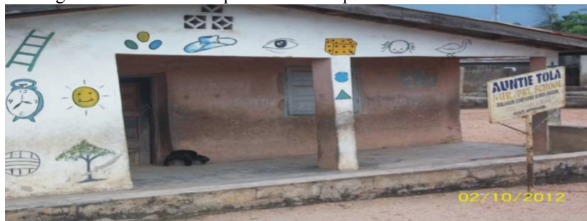
Plate 7: Condition of Educational Facility in the study area
