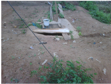
Plate 3a: An uncovered hand-dug well. Source: Field survey, 2012
