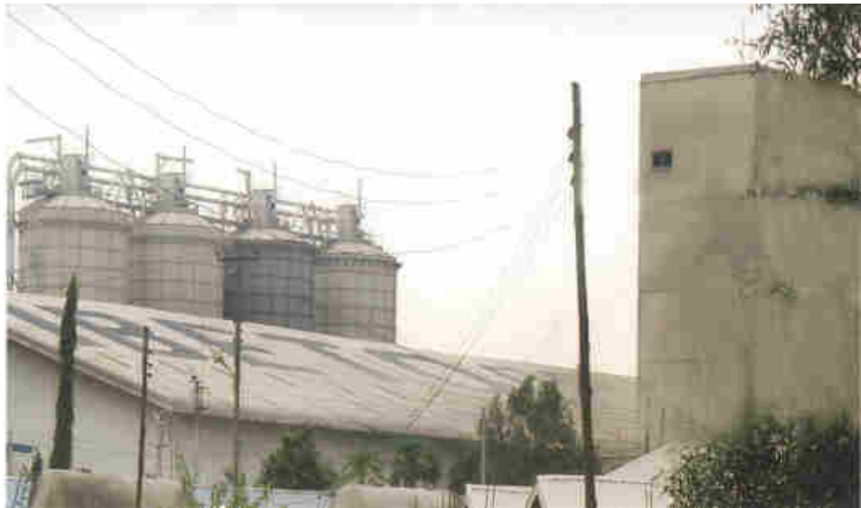
Figure 3: Premises of Cement Bagging Industry (Ibeto)
